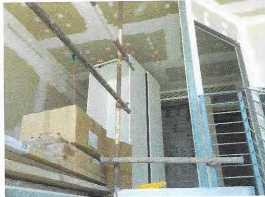
Loft – upper level
