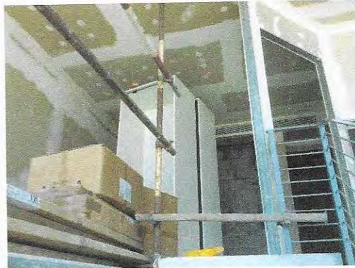
Loft – upper level
